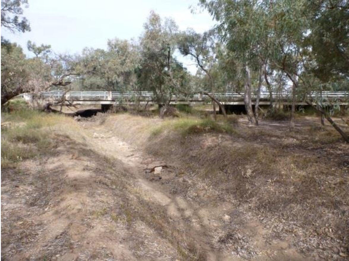
Fig A3-1. Calder Hwy Bridge
